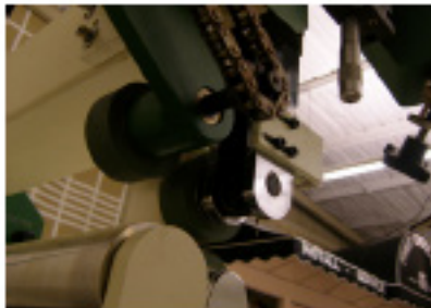
5. Remove the out puller cover and weld...
